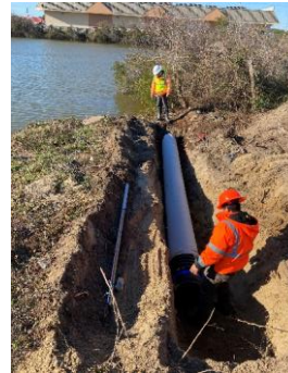
In the photo above, workers install the first 20' section of 15" drainage pipe from Virginia Dare Trail into the "turtle pond" between "Jolly Roger" and the movie theaters. This will relieve a frequently-flooded section of the road.
