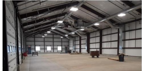
Photo above shows the interior of the New Solid Waste Building.
