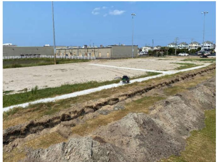
Looking northeast, trench in foreground is new storm drainage pipe for field in play area. New sidewalks run along south side of future play area and Splash Pad. Buildings in background are Dare Centre, north of site.
