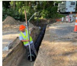
(Above) Checking pipe trench grade, 700 block of Cedar Drive.
