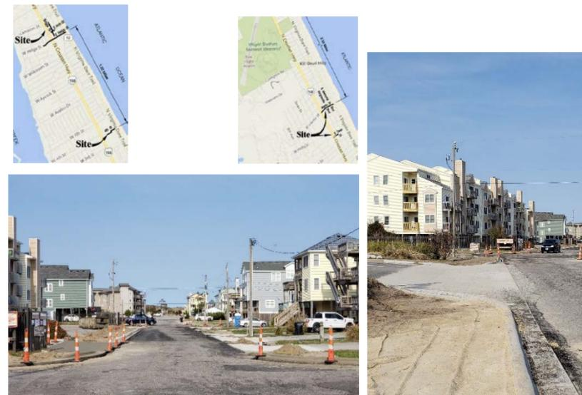
Both photos looking east along E. Martin St, new aprons on both sides of road, new curb and gutter on north end of road. Right photo is CVS entrance.
