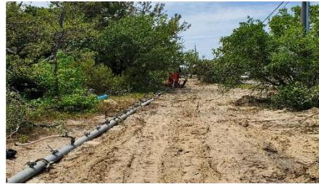
Photo above, looking westward toward Veterans Drive, 8" water main installation has been completed. The pipe at left is a well-point header, used to lower the groundwater table so that the pipe trench, nearly 4' deep, can be dry for proper pipelaying.
