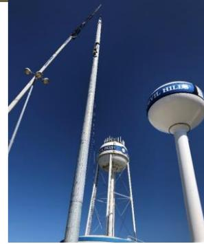
Photos above: [Left] Shows a climber guiding the top/6th section of new monopole cell tower into place; new water tank is at left, old ground storage tank at lower left. [Right] New tower (left, with crane) and new 400,000 gallon elevated water tank; in between are the old 200,000 tank (cell antennas on top) and, below, existing ground-level water storage tank.
